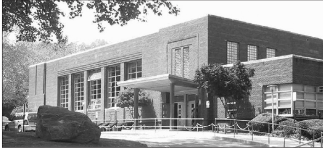
Saddle Rock School's auditorium will be improved and water-penetration problems addressed as part of the Capital Projects.
