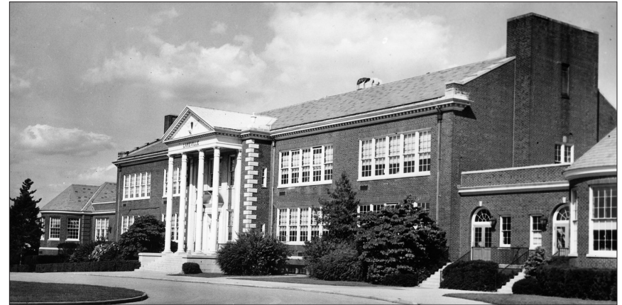
Lakeville School's roof will be replaced and the parking lot refurbished as part of the Capital Projects.
